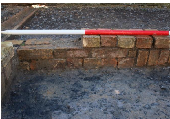
Figure 90: West yard, footing [0138] (facing north-east, PA2016_01_1039)
