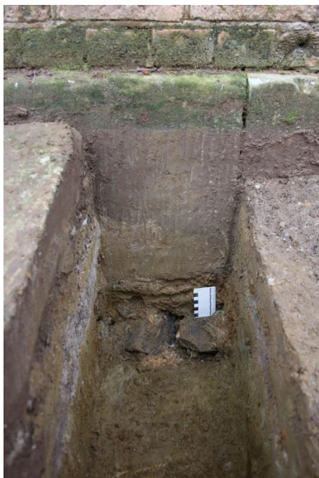
Figure 40: West yard, SS 2, showing Penitentiary footings [0002] (facing north-east, PA2016_01_1584)
