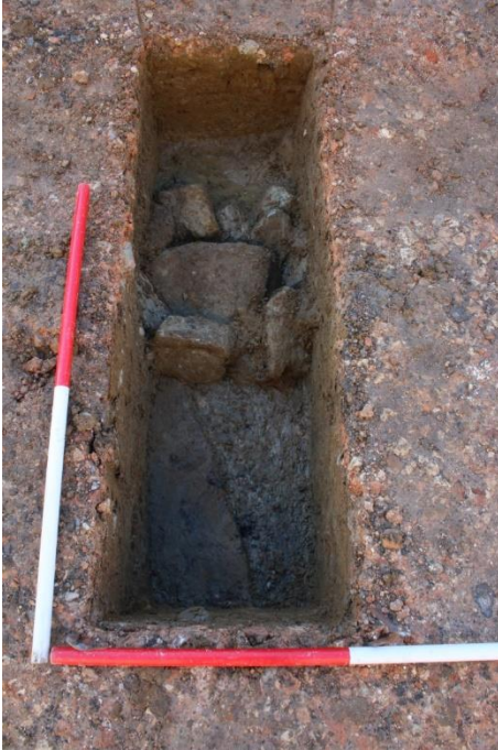
Figure 42: West yard, DS 6, drain [0554] (facing north-east, PA2016_01_1666)
