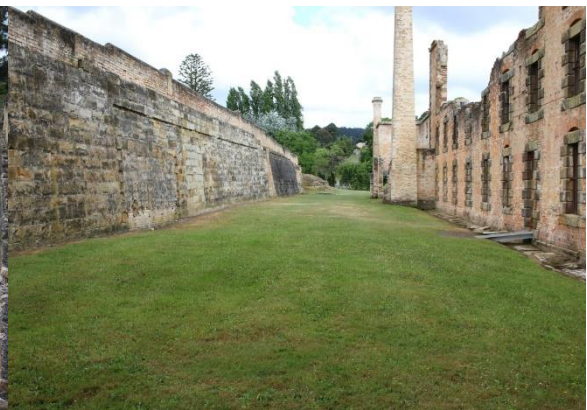
Figure 25: Penitentiary ablutions, pre-excavation (facing north-west, PA2016_01_0008)
