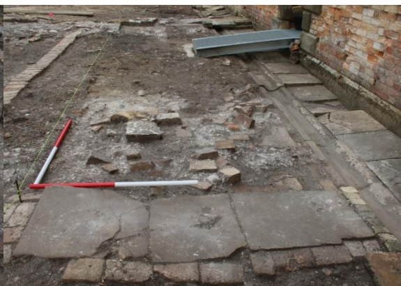
Figure 113: Day room, showing demolition debris at north end of space (facing north-west, PA2016_01_0296)
