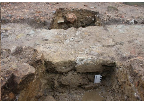
Figure 59: West yard, WS 2, showing depth of footing [0326] (facing north, PA2016_01_1502)
