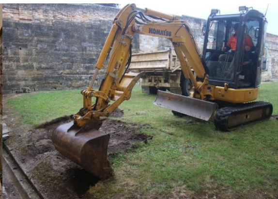
Figure 27: Penitentiary ablutions, mechanical excavation (facing west, PA2016_01_0097)
