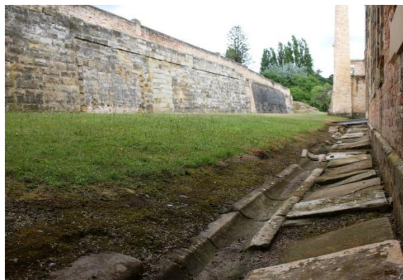
Figure 26: Penitentiary ablutions, pre-excitation (facing north-west, PA2016_01_0012)
