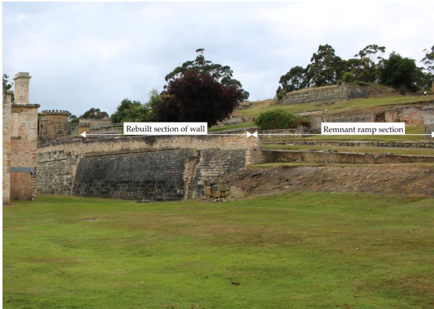
Figure 130: Showing area of excavation, with remnant section of 1830-ca.1855 ramp and the section of the Champ Street retaining wall rebuilt in ca.1855 (facing south)
