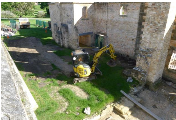
Figure 41: Penitentiary laundry, pre-excavation (facing north west, PA2016_05_0008)
