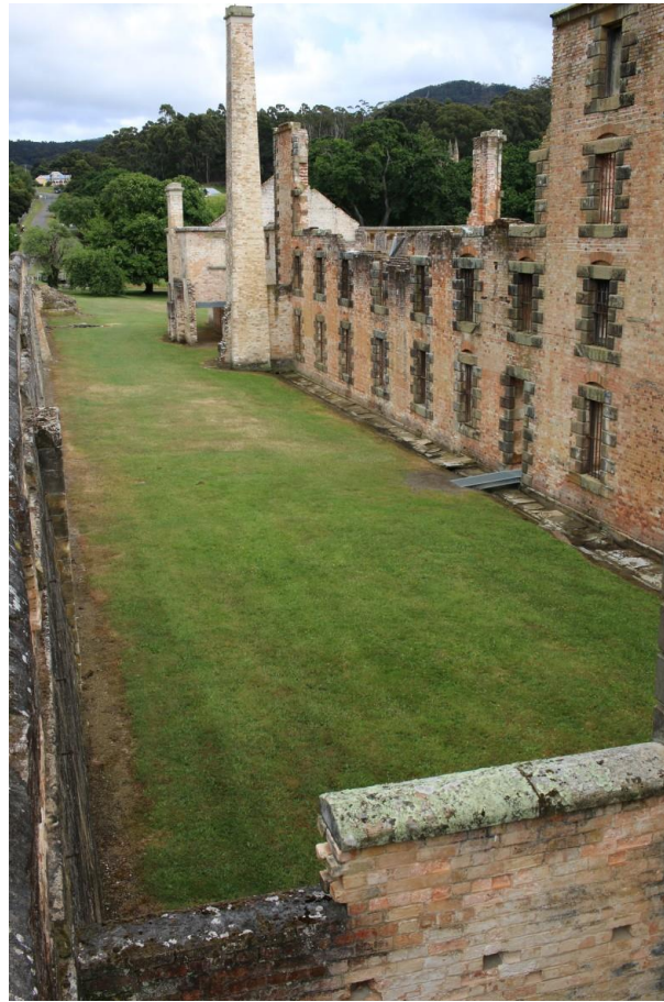
Figure 38: Penitentiary laundry and ablutions, pre-excitation (facing north north west, PA2016_05_0004)
