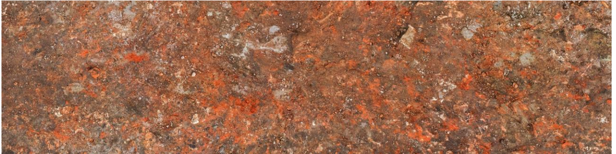
Figure 68: S5. Detail of crushed brick (0161) abutting chimney breast [0066]. Selection is 1.00m x 0.50m (facing north east, photogrammetry)
