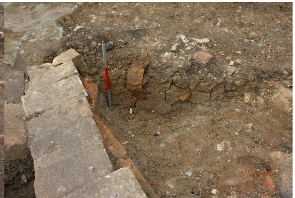
Figure 89: S1 (A1). Section through cut [0280] and clay (0277) at end of pipe (facing north east, PA2016_05_1344)
