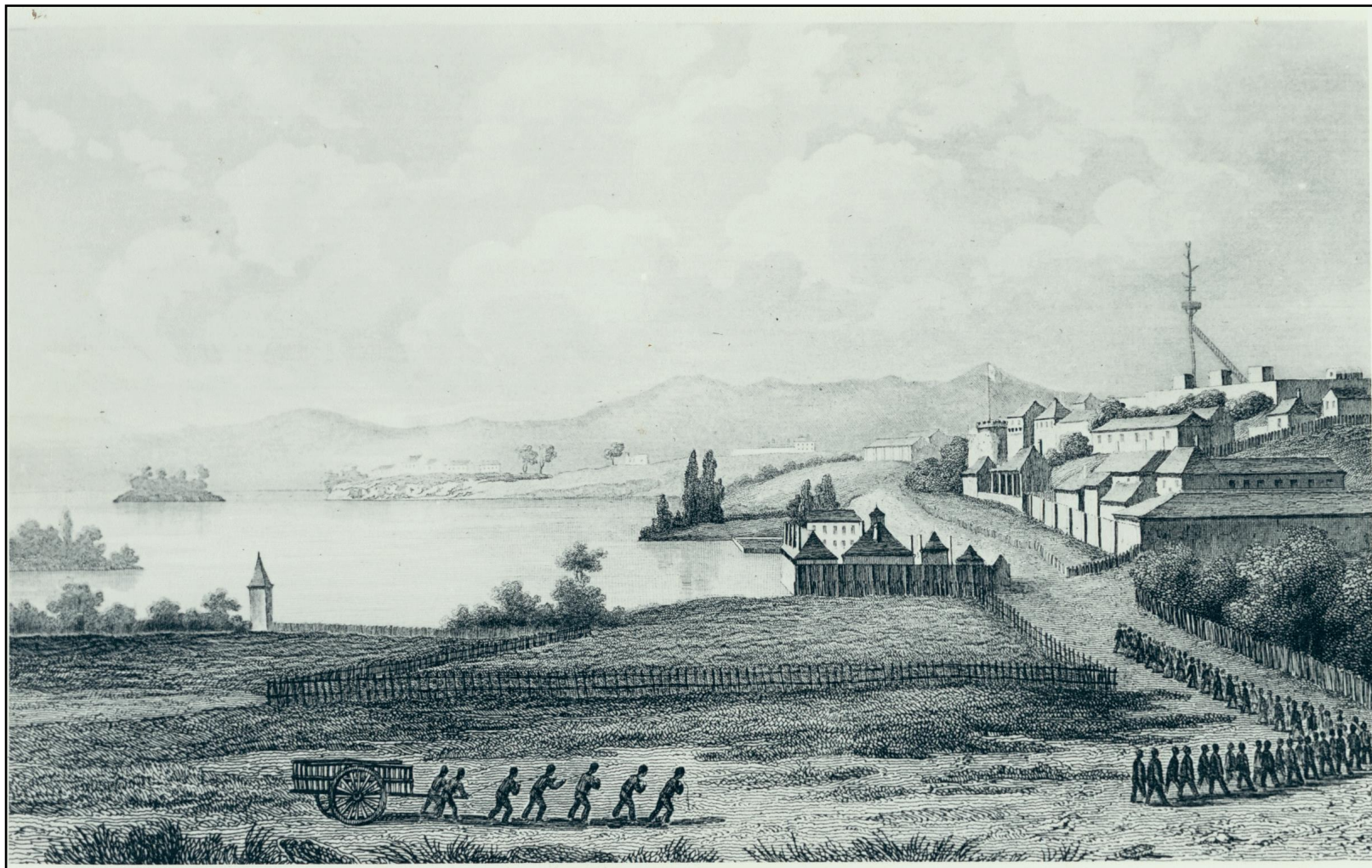
Figure 10: Illustration looking west. The workshops are shown in the foreground, with the Commissariat stores prominent behind (F.E.Paris, untitled, 1839, PAHSMA Collection, 'View from Scorpion Rock', #1366)
