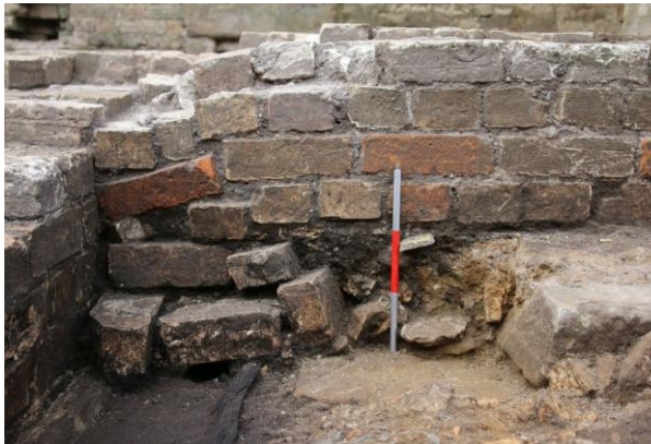
Figure 110: S9 (A2). Footing [0394] showing rough-built bricking [0220] above drain [0261] (facing north east, PA2016_05_0845)
