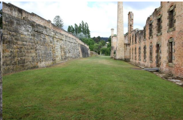
Figure 40: Penitentiary laundry and ablutions, pre-excitation (facing north west, PA2016_05_0008)
